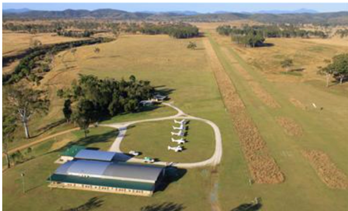
Old station runway and accommodation block
